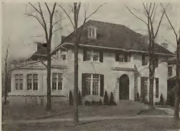
HOUSE OF C. F. MELLISH, DETROIT, MICHIGAN MACFARLANE, MAUL AND LENTZ, ARCHITECTS STUCCO ON INTERLOCKING TILE.
